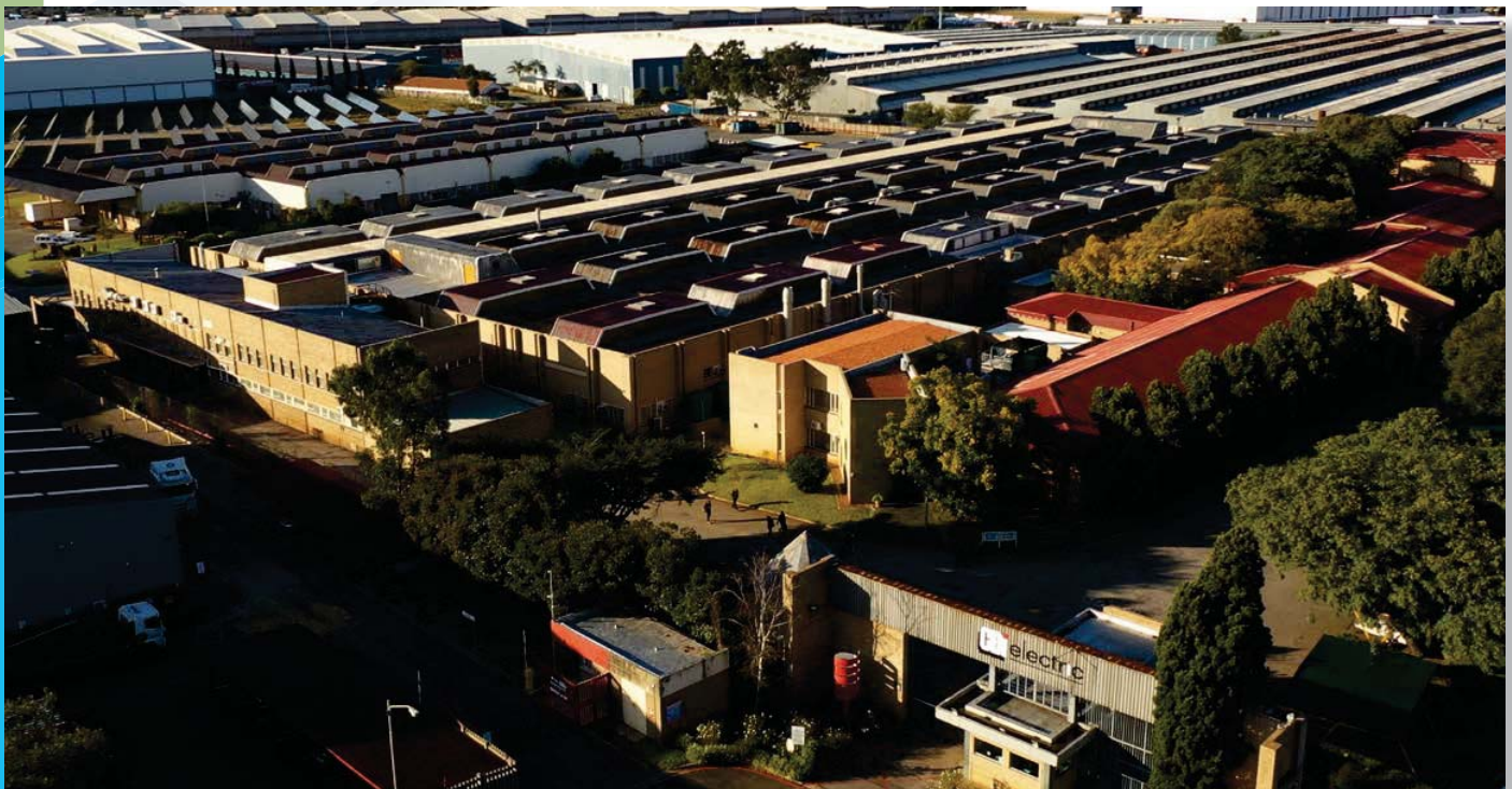
CBI-electric: low voltage at Elandsfontein, Johannesburg
